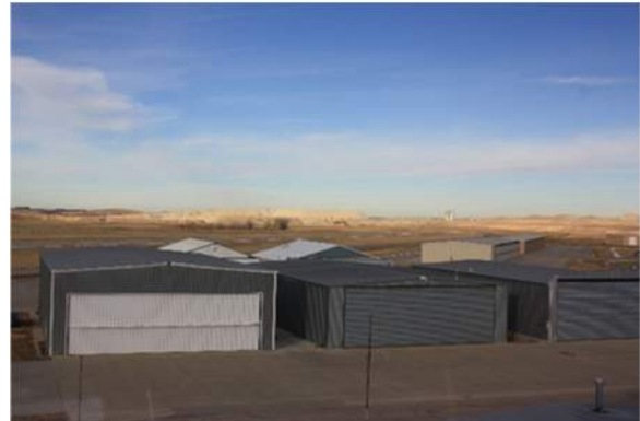
Figure 1-22. Private Hangars and T-Hangars
