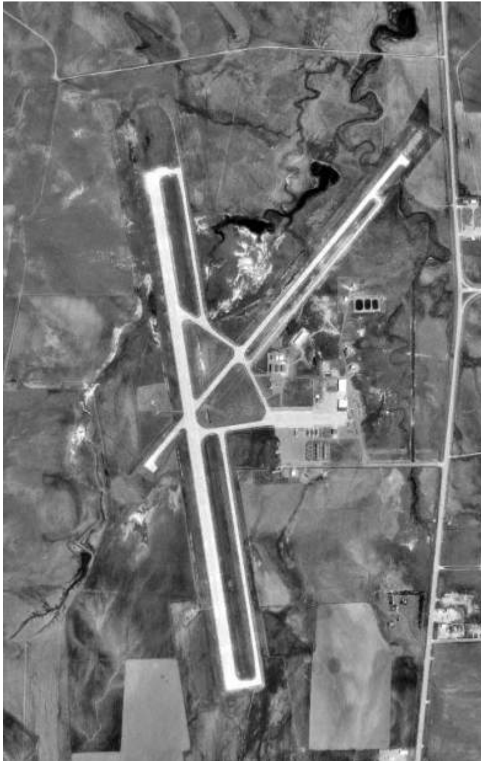
Figure 1-1. Gillette-Campbell County Airport, Google Earth Image from 1994
