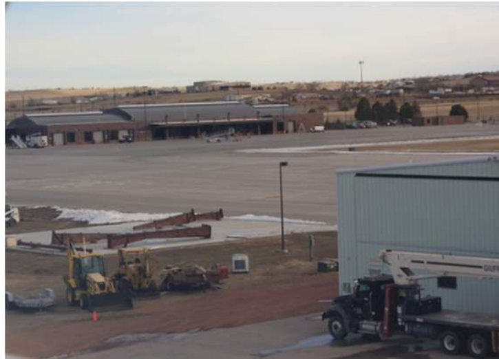
Figure 1-16. Commercial Apron view from the tower
