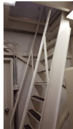
Figure 3-5. Existing Tower Access
