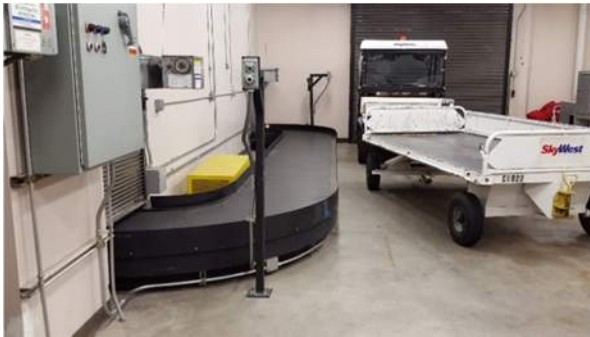
Figure 3-15. Baggage Claim Handling Area
