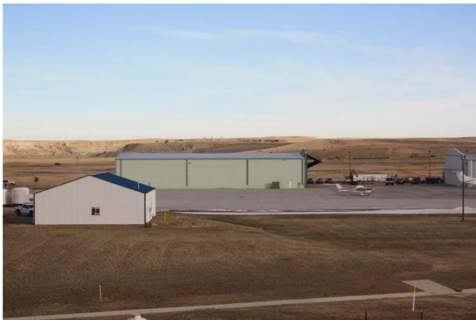
Figure 1-17. General Aviation Apron in front of the county hangar, view from the tower.
